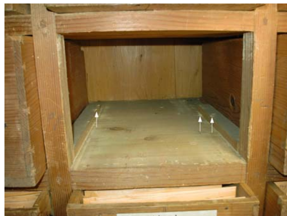
figure 3 A look into the shelf with an open drawer, the arrows indicating the damage caused by woodworm
