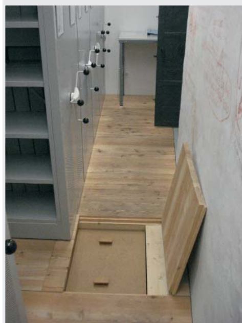
12 Access hatch from the archive room to the vaulted room.
