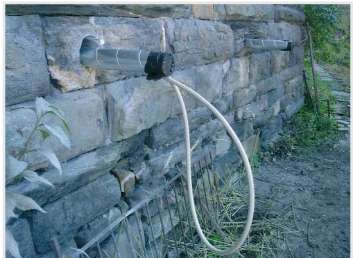
11 Front ventilation input and rear ventilation exhaust to the vaulted room beneath the archive room in the Marsöl Tower.
