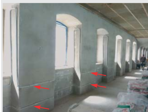
15 The wall heating pipes (arrows) prior to embedding in the window embrasures of the reading room and the archive office.
