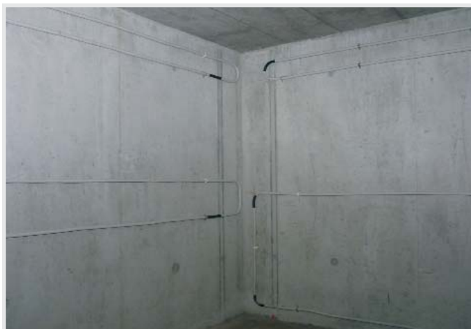
14 Prior to plastering the heating pipes mounted on the concrete walls (height 2.43 m).
